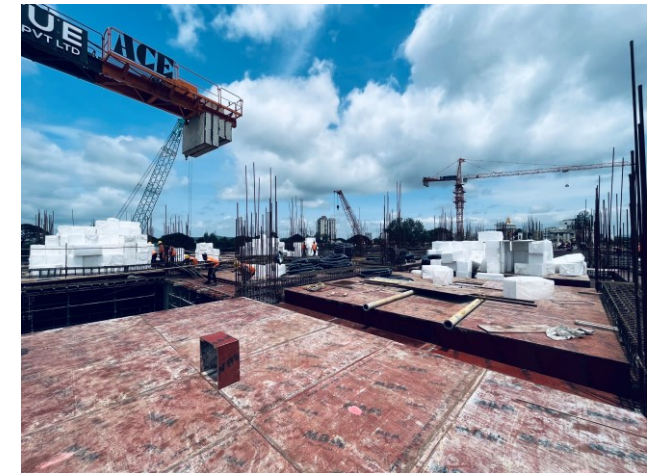
Pune Underground Metro
