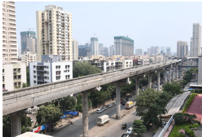
Mumbai Metro Line 6
