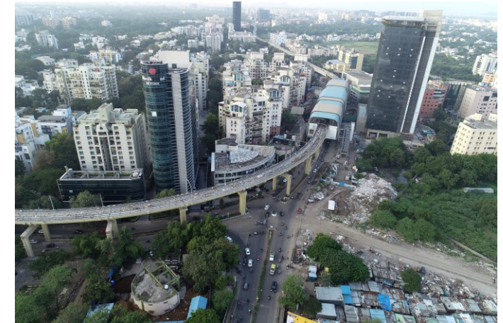
Pune Elevated Metro
