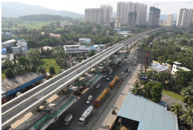
Mumbai Metro Line 4A
