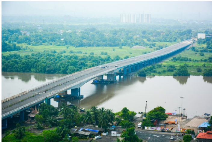
Motagaon Creek Bridge
