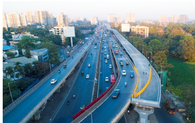
Chheda Nagar Flyover Part 1
