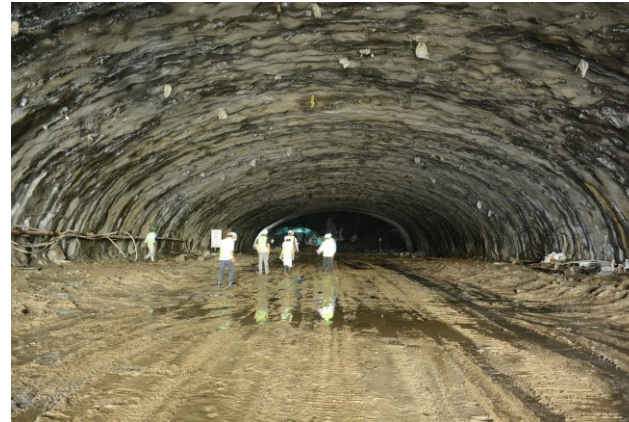
Vadodara Mumbai Expressway, IRCON
