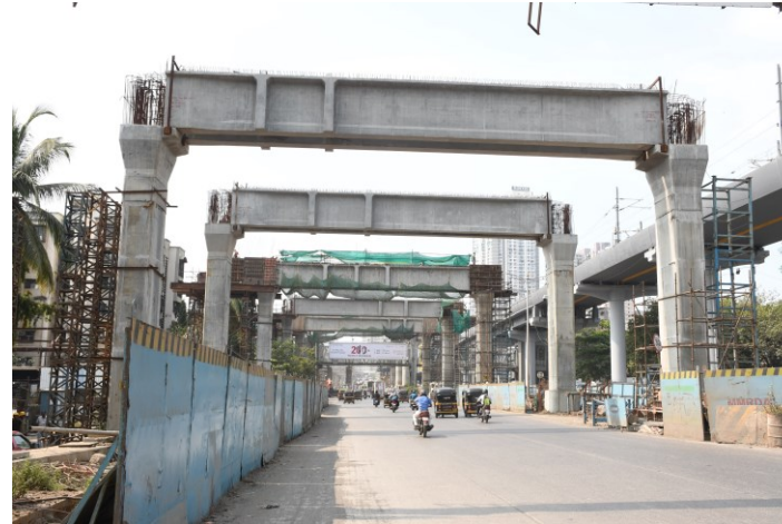
Mumbai Metro Line 9
