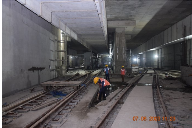
Mumbai Underground Metro Line 3
