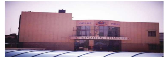
Police Station & Residential Quarters at Kondli, New Delhi for MHA, Delhi Police through RITES Ltd.
