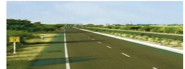
4 laning at Agra- Gwalior section, NH-2, in the State of Madhya Pradesh
