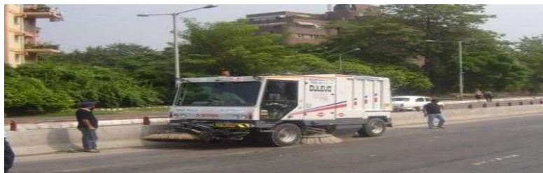
Comprehensive maintenance of Ring Road, Delhi
