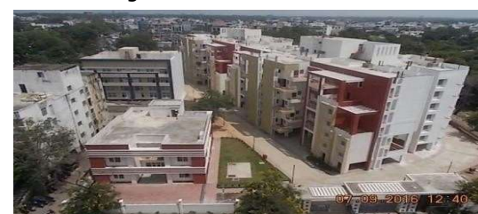
Construction of 92 flats at Mahadev Towers, Bhopal for MP Housing & Infrastructure Development Board
