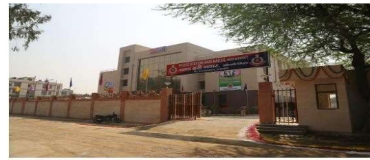
Construction of Police station & Residential Quarters, Hari Nagar, Delhi for MHA, Delhi Police through RITES Ltd.
