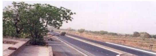
4 lane of km 41-51 of Agra Dholpur of NH-46 (earlier NH 3), in the state of Rajasthan
