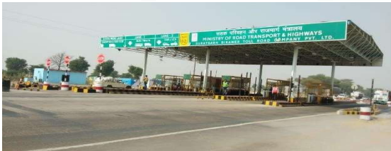
Development & Operation of Bikaner-Suratgarh Section of NH-62 (earlier NH-15) in the state of Rajasthan
