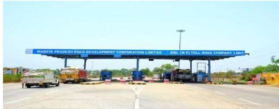
Strengthening, Widening, Maintaining and Operating 18.303 kms Waraseoni-Lalbarra Road in the state of Madhya Pradesh
