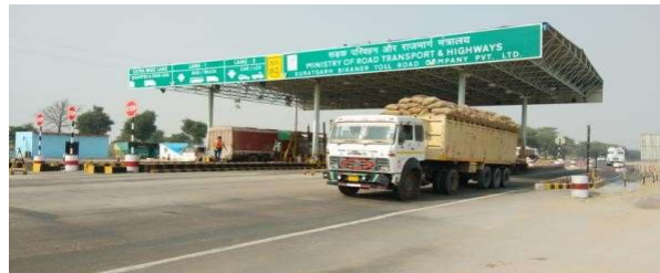
Development & Operation of Bikaner- Suratgarh Section of NH-62 (earlier NH-15) in the state of Rajasthan
