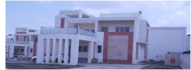
Construction of Director, QIP Centre & Accom. for School of Planning & Architecture at Bhopal
