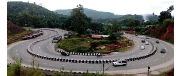
Widening & Strengthening of existing National Highway from 2 lane to 4 lane of Sonapur to Guwahati section of NH-115 (earlier NH 37)
