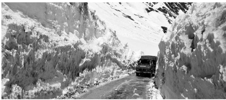
The cost of the proposed Shingo La tunnel project is expected to be similar to that of Zojila tunnel project. The lowest bidder for Zojila had quoted ₹4,509 crore
