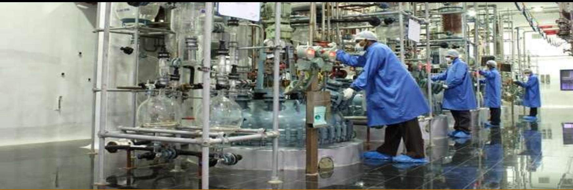
Glass Lined Reactors in Intermediate Area
