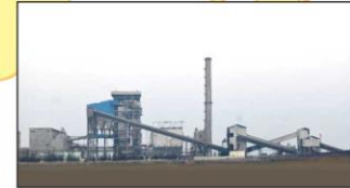
CAPTIVE POWER PLANTS (143 MW, MULTI-FUEL)
