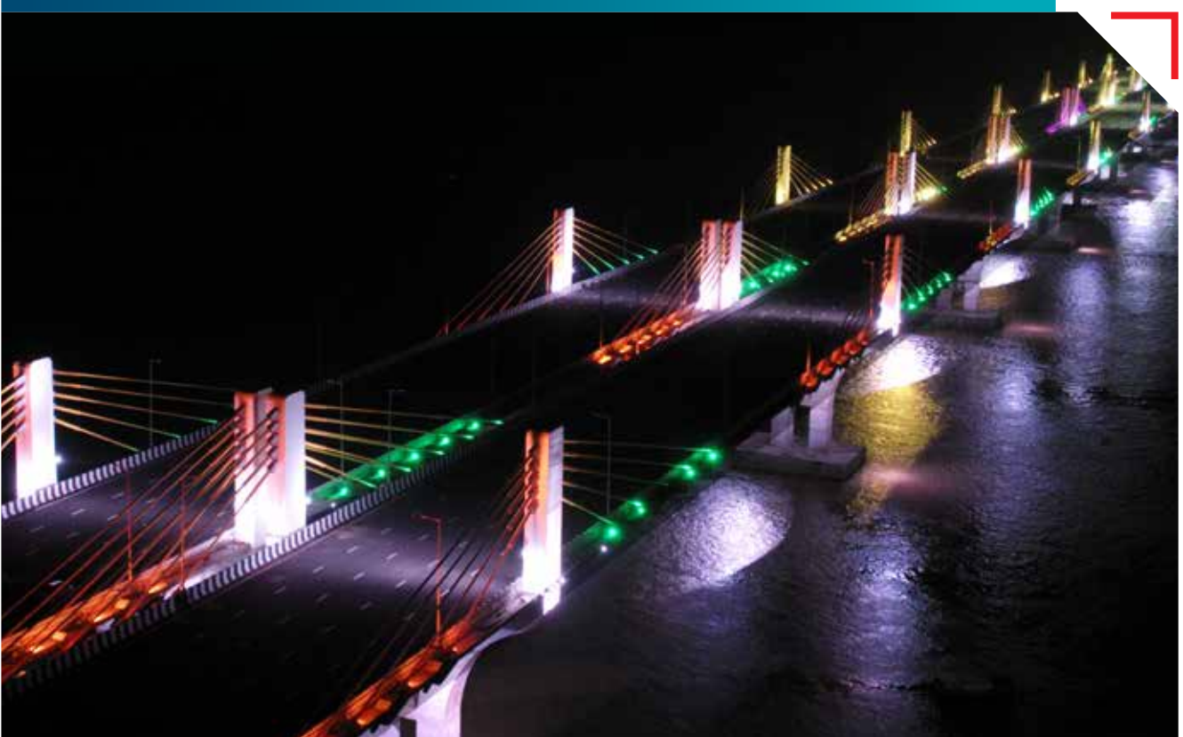
NARMADA BRIDGE FACADE
