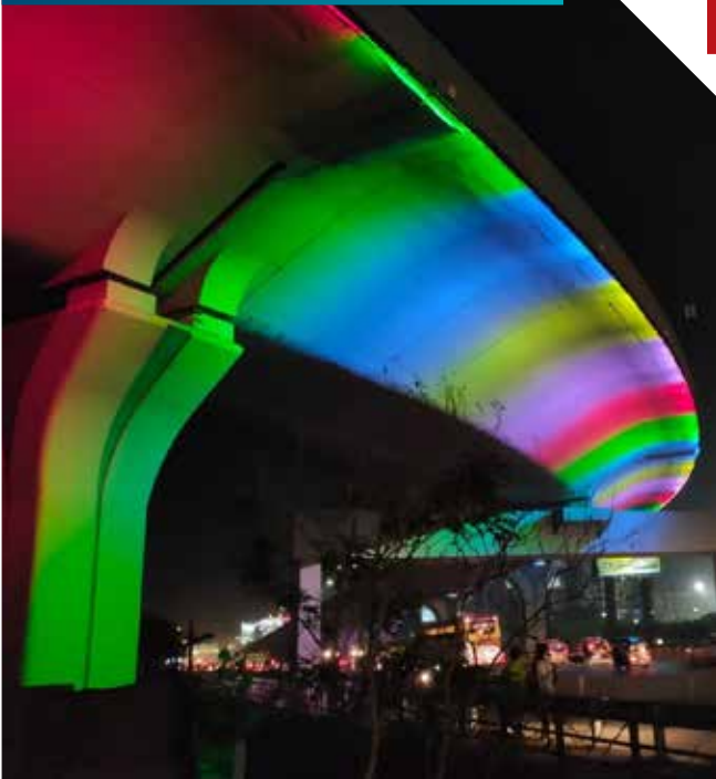
KURLA BRIDGE EXTENSION
