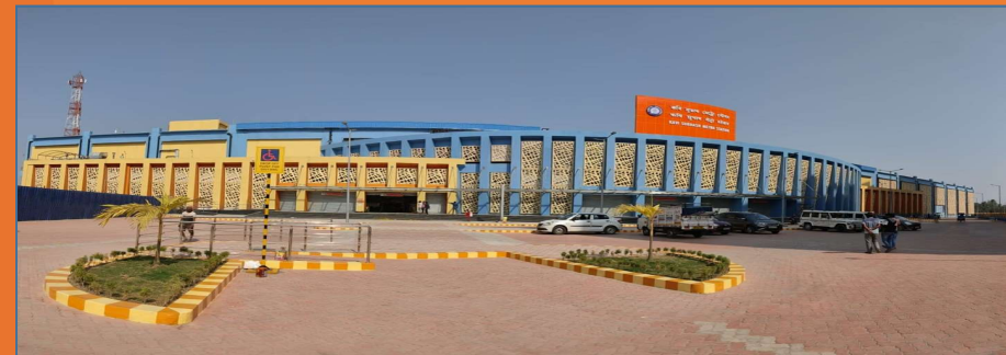
Kolkata metro station building in West Bengal
