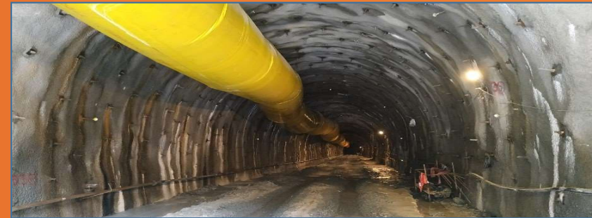
Sivok Rangpo railway tunnel in West Bengal and Sikkim
