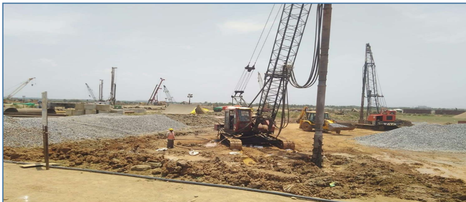
Piling and Ground improvement work in Odisha
