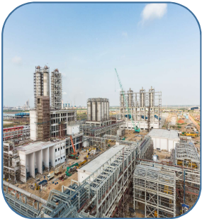
INDUSTRIAL STRUCTURES AND BUILDINGS
