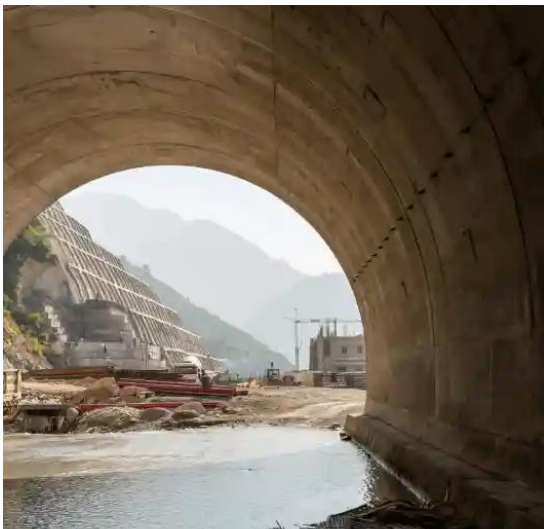
Tunnel T - 5, KRCL
