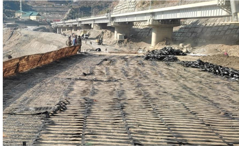
RE Wall, Sumber, HCC
