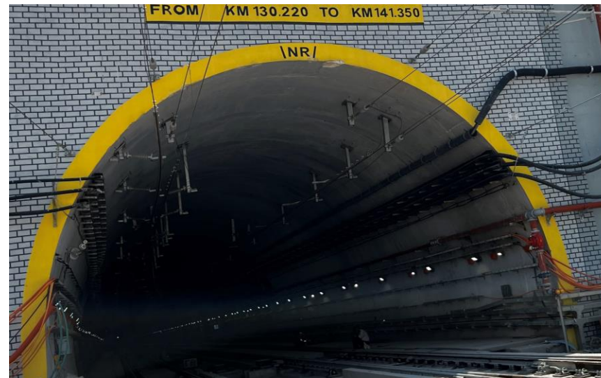
Tunnel T - 41, KRCL
