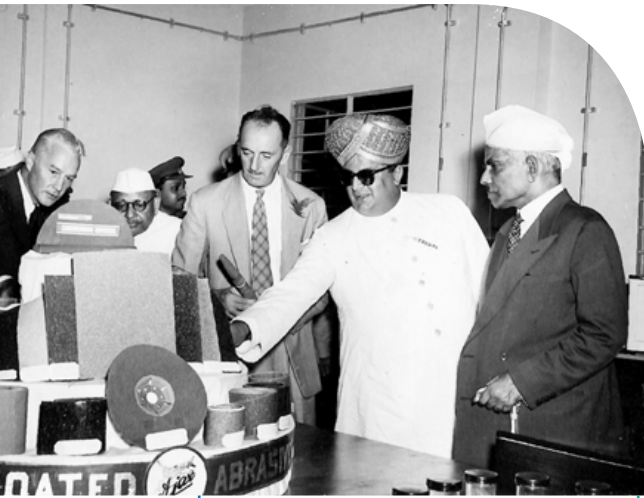
1955: Jayachamarajendra Wadiyar, the Maharaja of Mysore, inaugurates CUMI's Coated Abrasives plant
