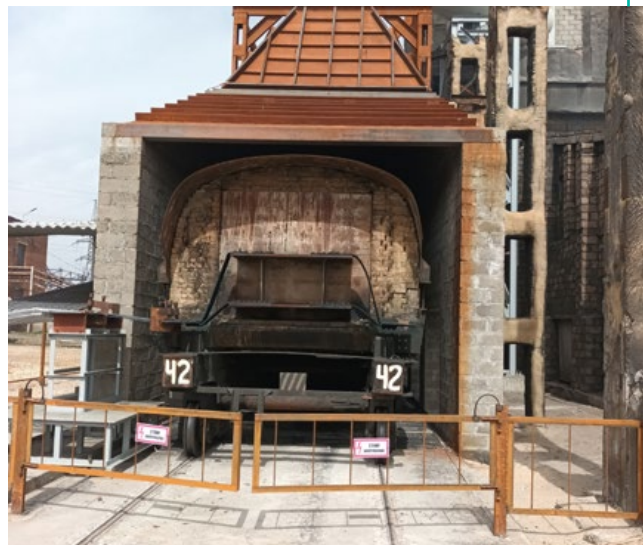
The newly commissioned Fusion Cell
