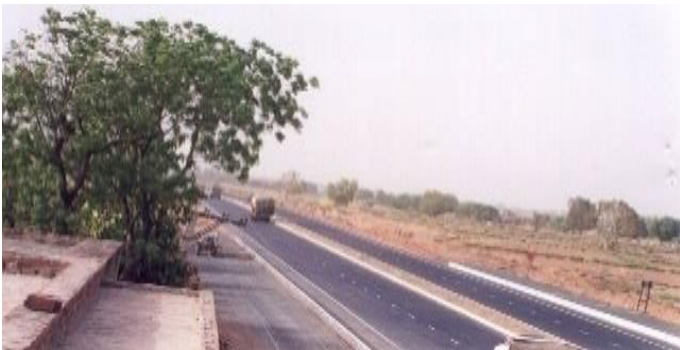
(Four lane of km 41-51 of Agra Dholpur of NH- 46 (earlier NH 3), in the state of Rajasthan)
