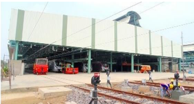
(Construction of Metro rail depot, Kalindi Kunj, New Delhi)
