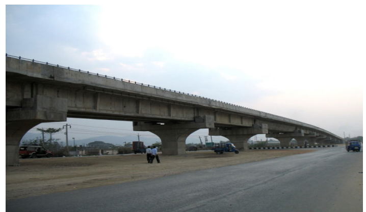
(Widening & Strengthening of existing National Highway from 2 Lane to 4 Lane from Km 183.000 to 163.895 of Sonapur to Guwahati Section of NH-115 (earlier NH-37 in the State of Assam on EW-II under program of NHDP Package AS-03)
