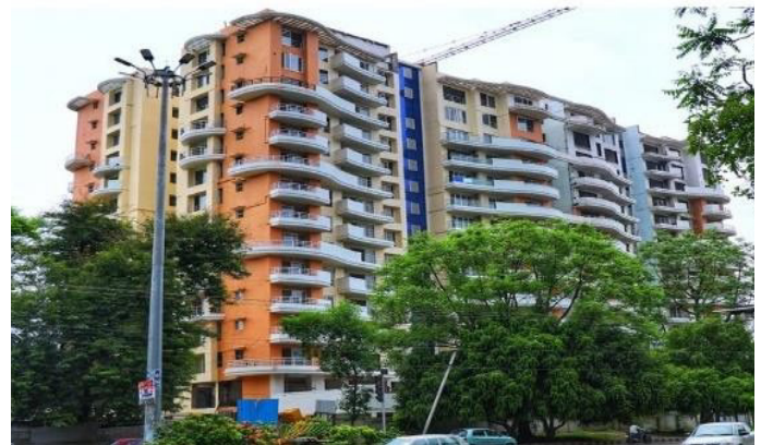
(Construction of 96 flats at Tulsi Tower, Bhopal for MP Housing & Infrastructure Development Board)
