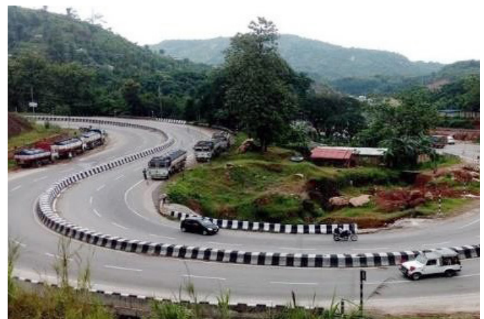
(Widening & Strengthening of existing National Highway from 2 lane to 4 lane of Sonapur to Guwahati section of NH-115 earlier NH-37 )
