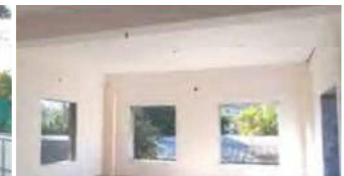
Classroom construction WIP at Marunji, Pune
