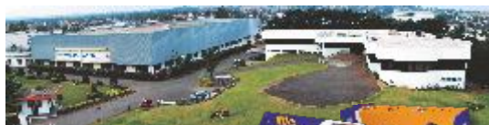
Menon Bearings plant at Kolhapur,
