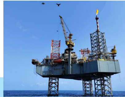
KGB- Offshore Installation at B-80 Site
