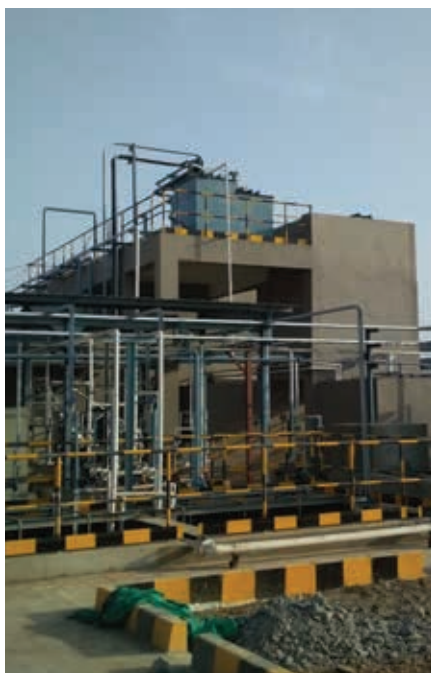
Upcoming Resin manufacturing facility of PPG-AP at Dahej.
