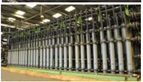
110 MLD SWRO (Desalination) Plant, Nemmeli, Chennai, India India's largest operational desalination plant till date
