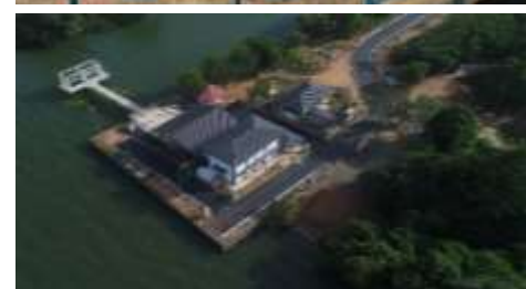
32 MLD Drinking Water Treatment Plant, Dambulla, Srilanka Integrated water supply scheme with transmission, distribution and water treatment
