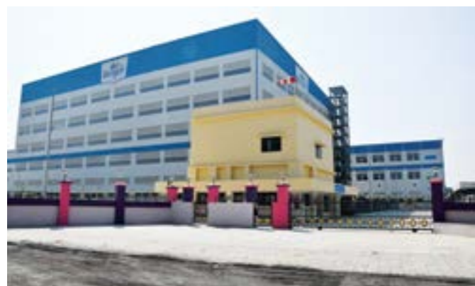
New Sandila (Uttar Pradesh) plant
