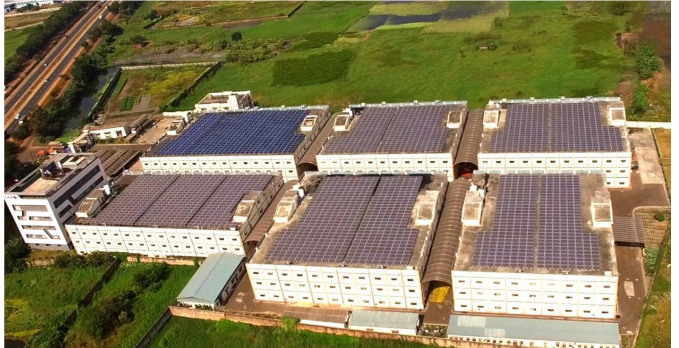
Rooftop solar power plant at Dankuni unit
