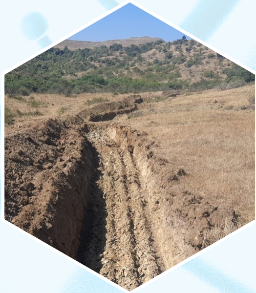
Ongoing Soil and water conservation work
