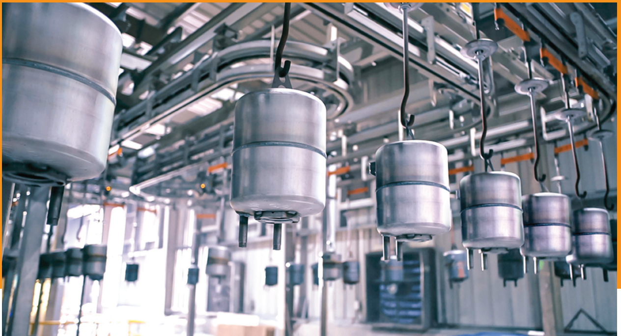
Fully automated vitreous enamel coating line at the water heater factory, Sikkim
