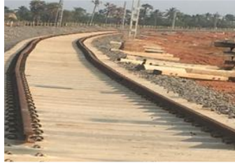
GDV-MTM 37 ,DOUBLING & ELECTRIFICATION WORKS , RVNL
