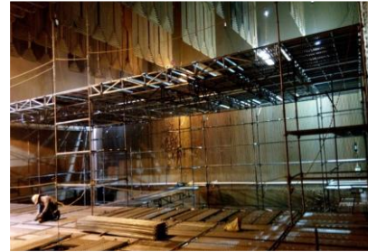
CUPLOCK SCAFFOLDING ERECTION 800MW,MUNDRA
