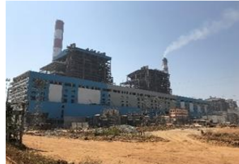
2X660 MW IBTPS, STRUCTURE & STG, BANHARPALLI, BHEL
