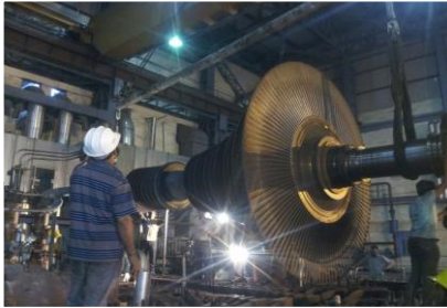
CAPITAL OVERHAULING OF TURBINE 63MW, SV POWER , KORBA - ROTOR LIFTING-3
