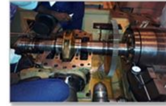
228MW, STEAMTURBINE,SABIYA, KUWAIT, MAIN OIL PUMP OVERHAULING
