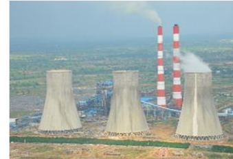
2X660 MW JTPP, BOILER,ESP & CP, JHAJJAR, STEPC (COMPLETED)
