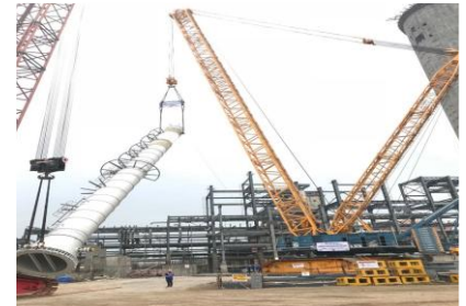
UREA REACTOR TANK INSTALLATION AT RAMAGAUNDAM, TELANGANA
