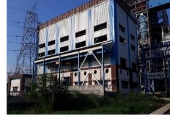
1X500MW, FGUTTP, CIVIL, STRUCTURAL AND ARCHITECTURAL WORK FOR BTP, BOP & CHP, UNCHAHAH, NBPPL
