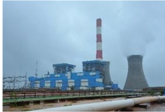
2X600MW TPP, BOILER & STG, MANGALORE, LANCO (COMPLETED)
