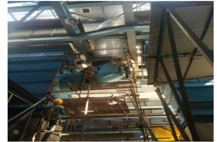
MSH LINE MODIFICATION, 600 MW SINGARENI
