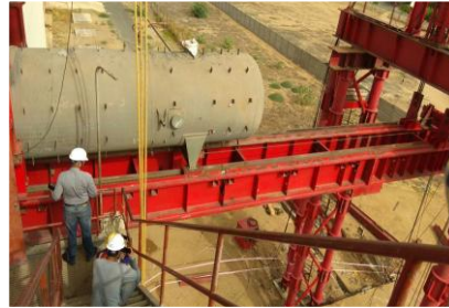
HP HEATER REPLACEMENT 800MW ,CGPL MUNDRA2
