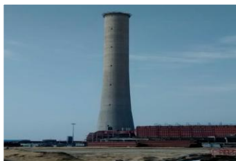
1X500 MW, FGUTTP, CIVIL, STRUCTURAL AND BOP & CHP, UNCHAHAH, NBPPL
