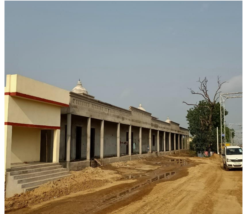
Station Building in Final Stage at Alal station
