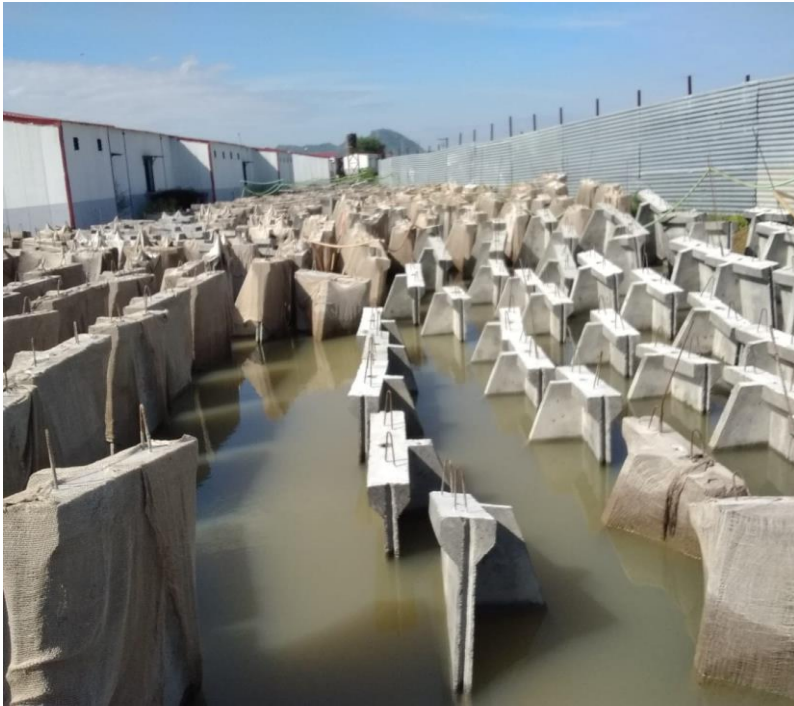
Platform Wall Curing
