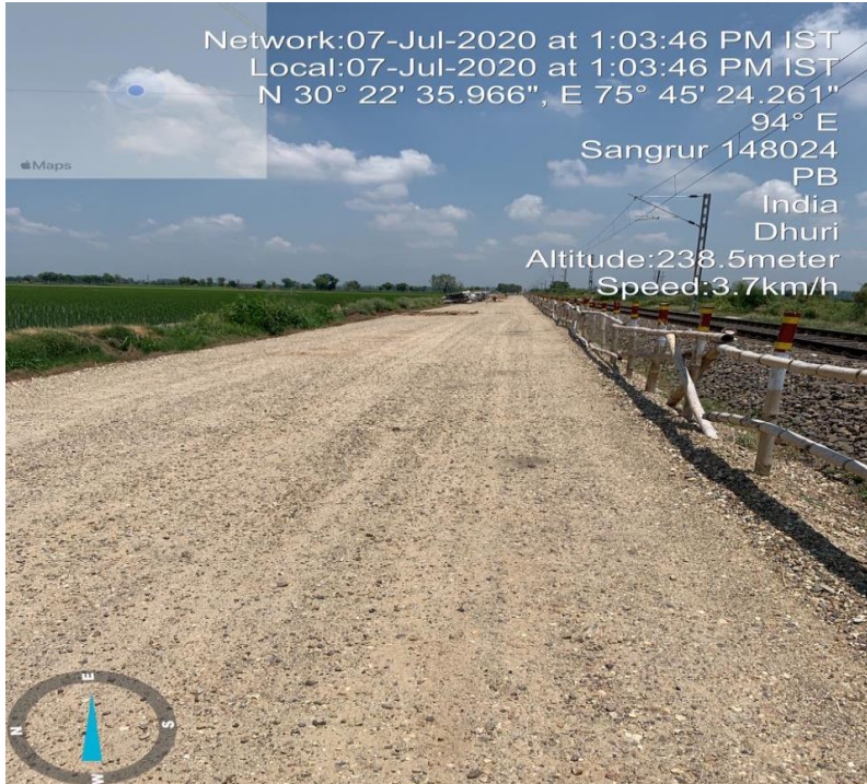
Blanket 3 rd Layer in progress at Ch. 88+400
