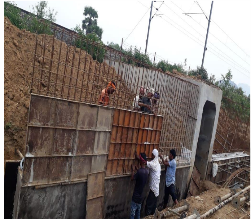
MNB 140 Retaining wall (WIP)
