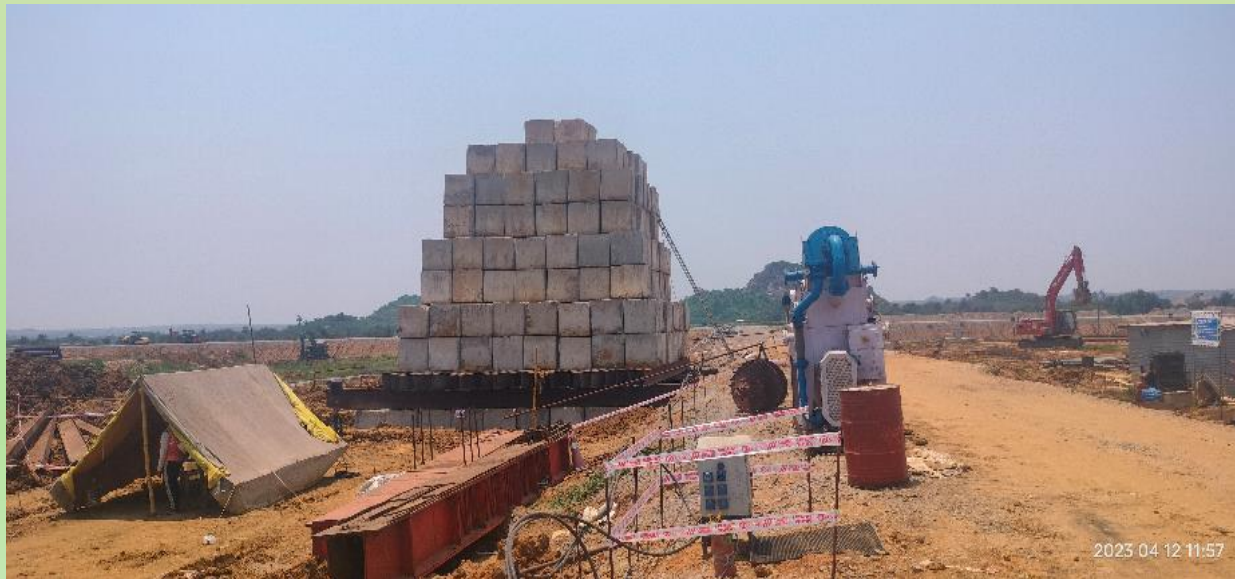
VERTICAL PILE LOAD TEST
