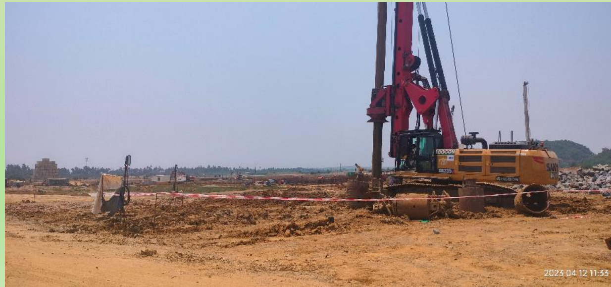
WORKING PILE IS IN PROGRESS AT PB-03
