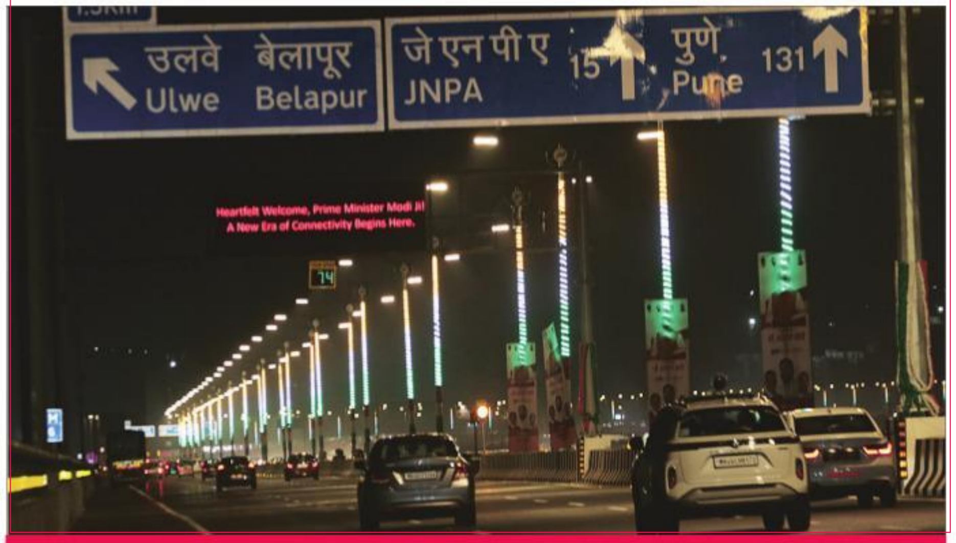
The Mumbai Trans Harbour Link, formally named Atal Bihari Vajpayee Sewari-Nhava Sheva Atal Setu, was opened to the public on Saturday. Prime Minister Narendra Modi on Friday inaugurated the 21.8-km long bridge, the longest in the country.
