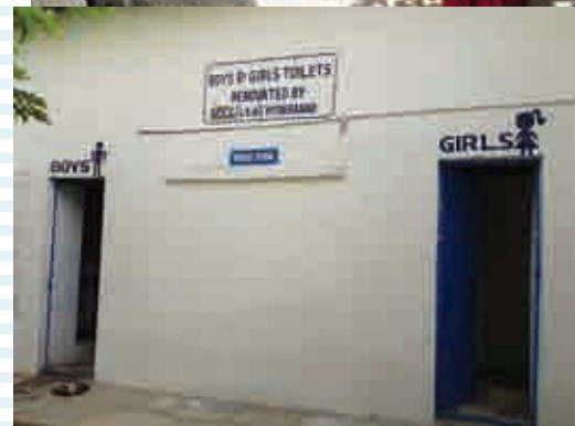
Toilets constructed in the School at Tandur, Telangana under CSR Initiative
