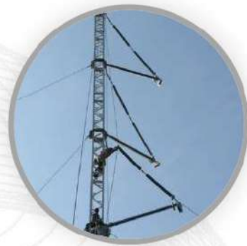
Emergency Restoration Systems (ERS) Supply and Installation
