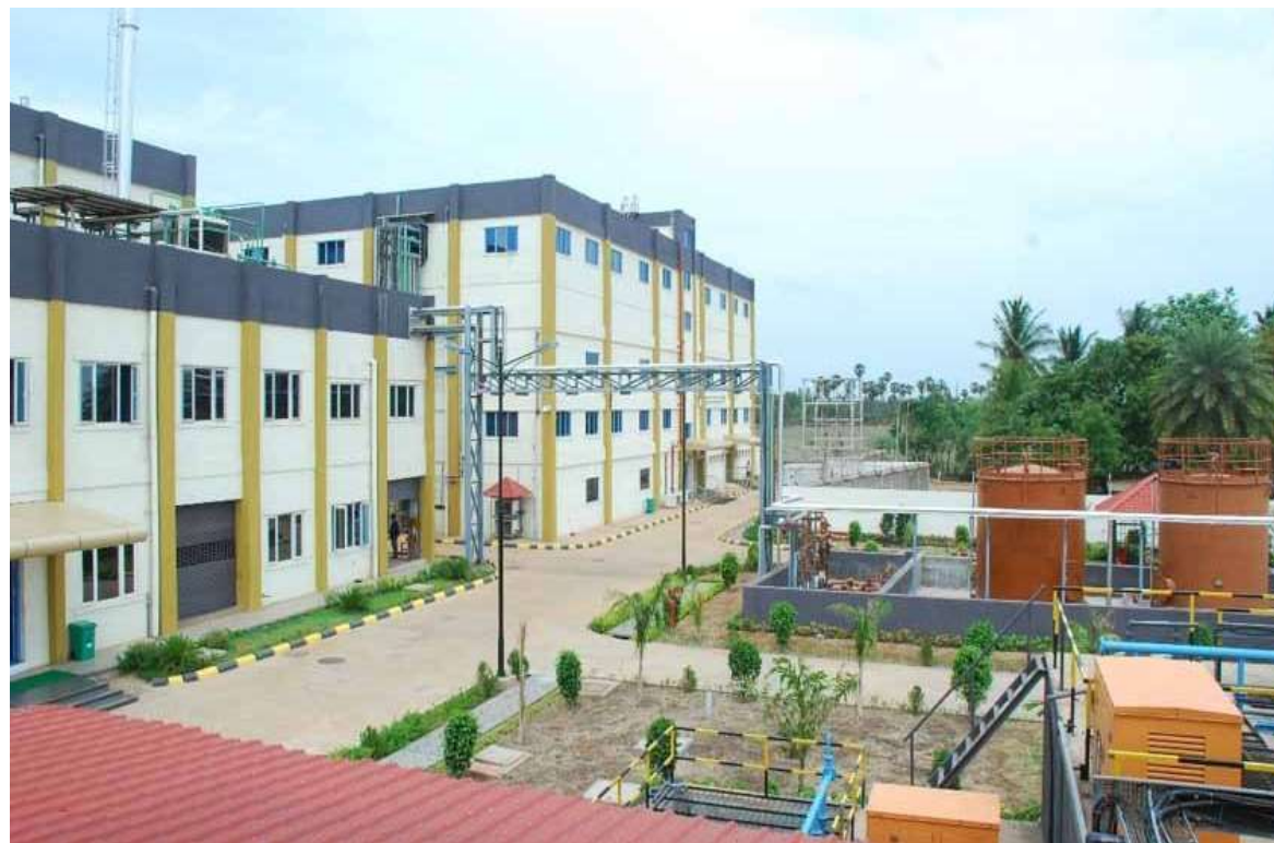
CP-IV plant at Gummidipoondi, Chennai
