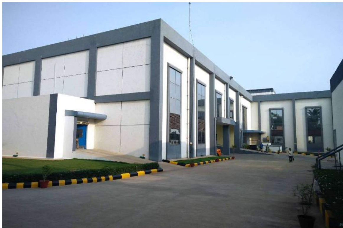
CP-I plant at Suthukeny, Puducherry
