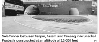
Sela Tunnel between Tezpur, Assam and Tawang in Arunachal Pradesh, constructed at an altitude of 13,000 feet
