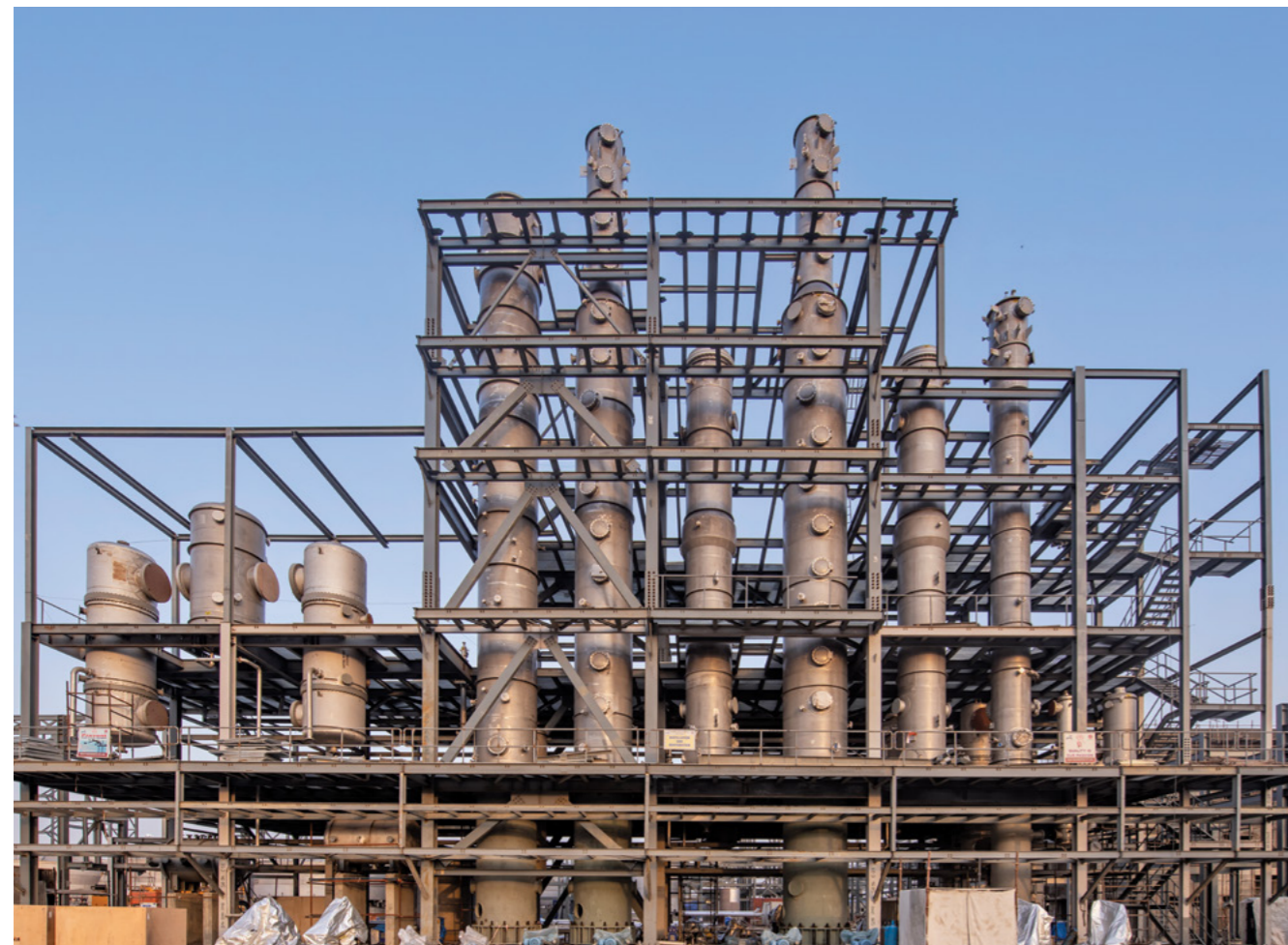
Upcoming 2G Ethanol plant at Panipat
