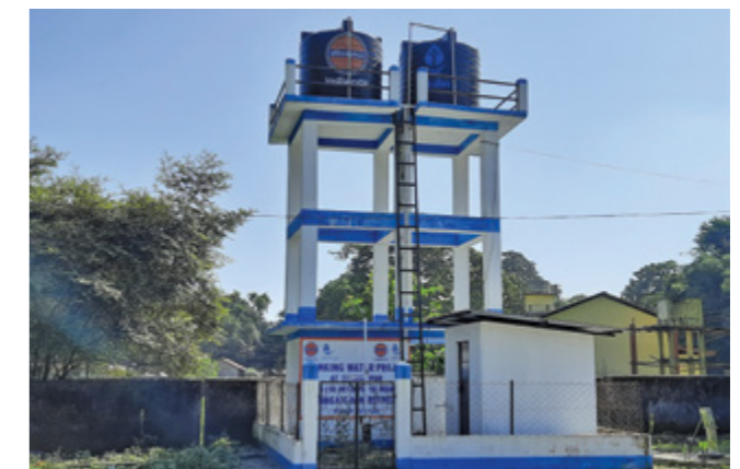
Drinking Water Project, Bishnupur, Bongaigaon in Assam
