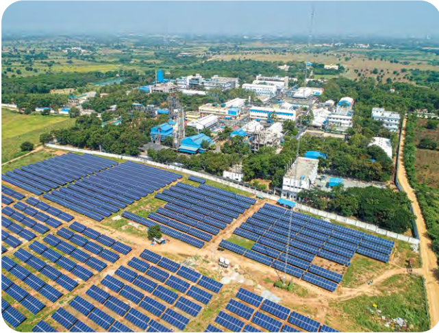
Aerial view of the solar power plant at our Mekaguda facility
