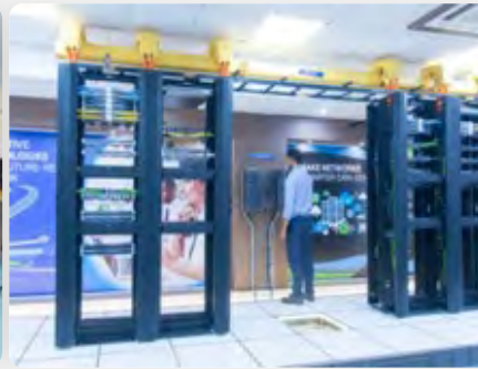
Optical Fibre Cables Design Lab, Silvassa
