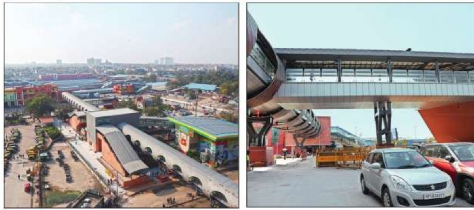
CONNECTING PEOPLE: This skywalk is an extension of the foot overbridge inside the railway station
