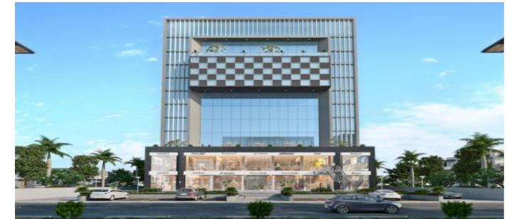
Motilal Oswal Tower - Ahmedabad
