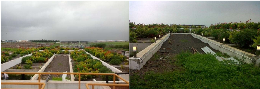
Mahindra Vehicle Manufacturers Ltd., Chakan MIDC (750 CMD ETP using Phytorid Technology)
