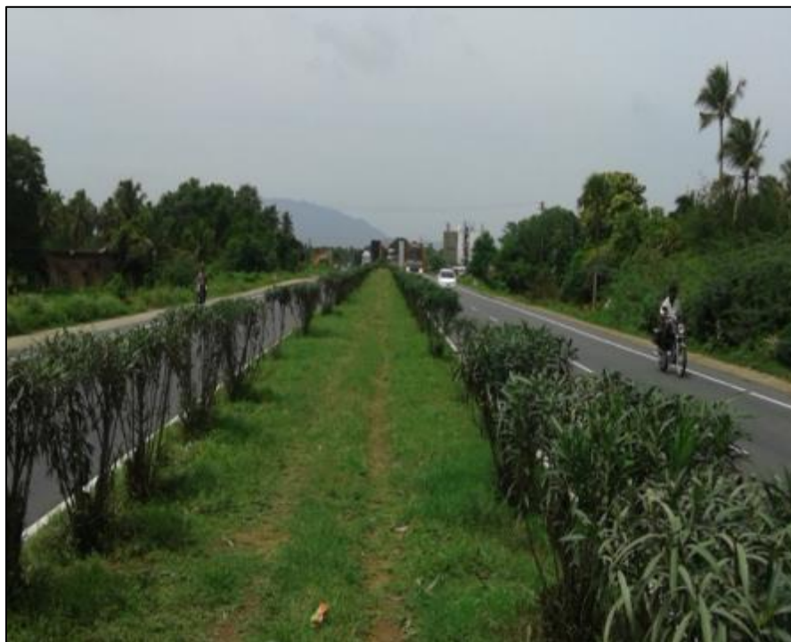
Figure 8-4 General Project Condition
