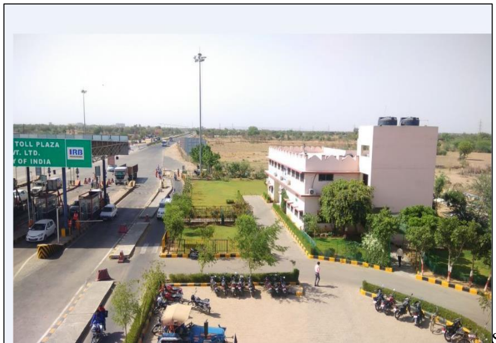
Figure 8-4 : Toll at Barkheda
