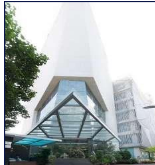
CCIL Bhavan Phase I : Upto 6 th floor
