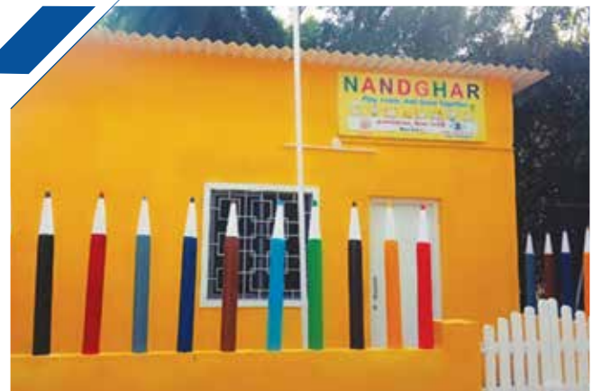
Renovation of school at Mandva, Gujarat
