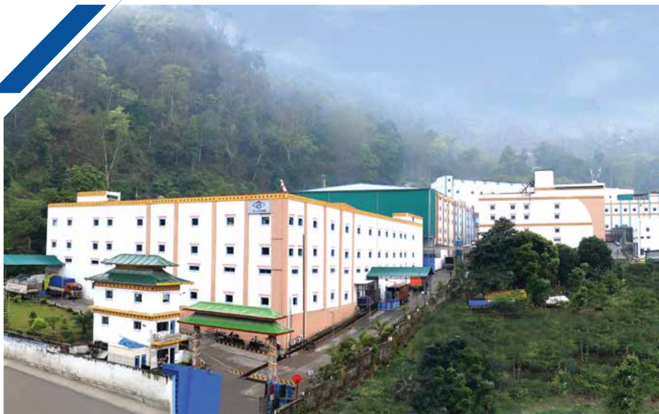
Company's manufacturing facilities in Sikkim (India)
