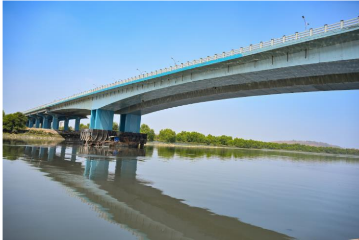
Motagaon Creek Bridge
