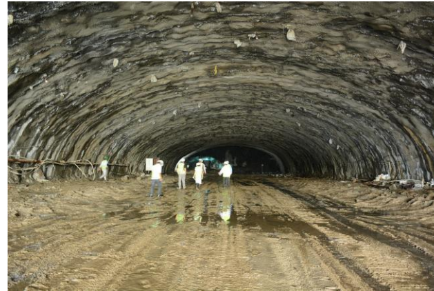
Vadodara Mumbai Expressway, IRCON
