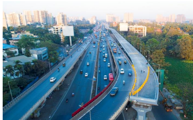
Chheda Nagar Flyover Part 1
