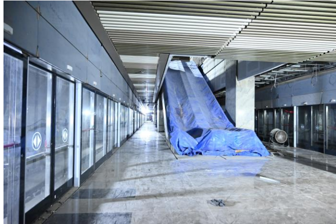
Mumbai Underground Metro Line 3
