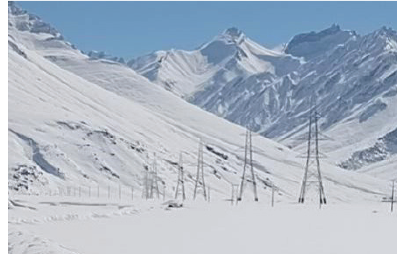
220kV Single Circuit Transmission Line from Drass to Padum on Double Circuit Tower at Kargil, Ladakh being implemented by RECPDCL
