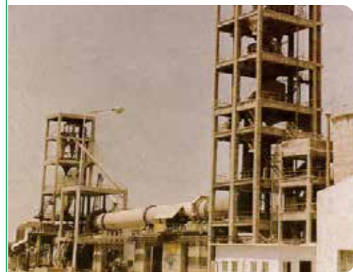
Plant commissioned with 200 TPD kiln four-stage preheater technology.
