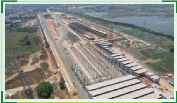
Drone Photo of Depot at Poonamalee, Chennai Metro Project
