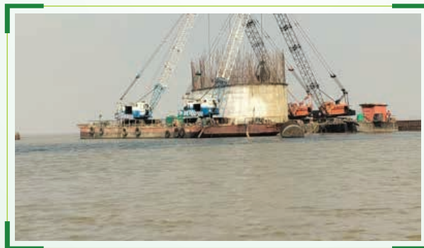
Well Foundation in Progress
