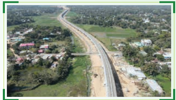
Viaduct, Agartala Akhaura Rail Link Project
