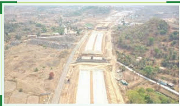
Areal View of Bhoj End Road Work
