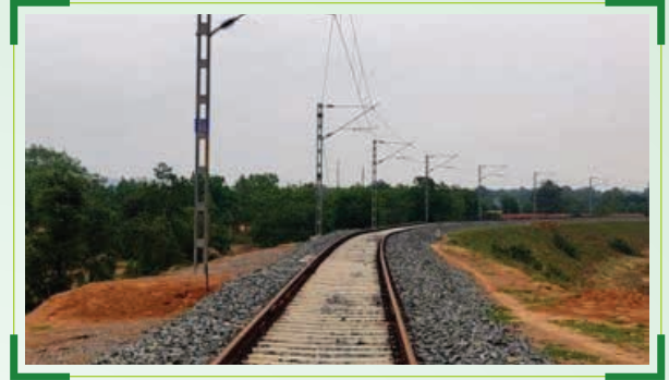
OHE Work in Korichhapar to Dharamjaigarh Section
