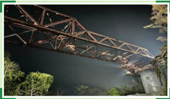
OWG Erection is in progress at Br. 02, Sivok Rangpo
