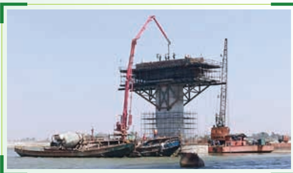
Casting of Pier Cap
