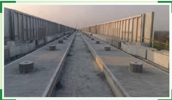
RC Track Bed Works on Viaduct at Ch. 237 Km, MAHSR T-2
