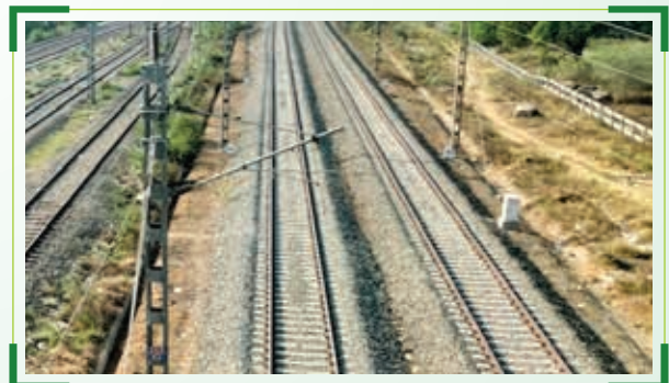
Completed Rail Formation Section at Vedchha, DFC Project
