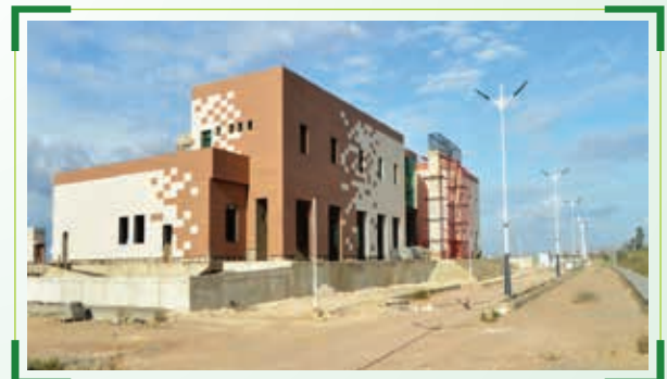
Relizane Railway Station, Algeria
