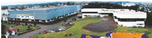
Menon Bearings plant at Kolhapur,
