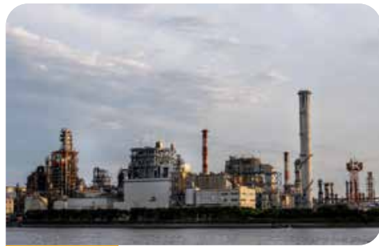
Primary & Secondary structures for boilers & turbine generators
