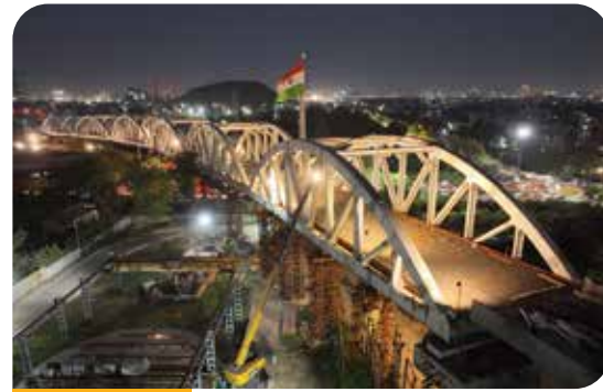
Structures for roads & bridges
