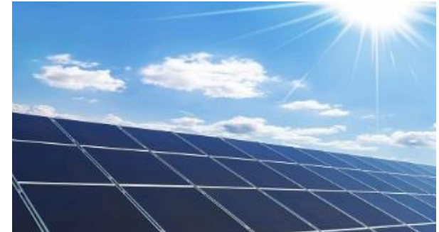
Signed first Onsite Solar Power Purchase Agreement 7.14 MW for Rabriyawas
