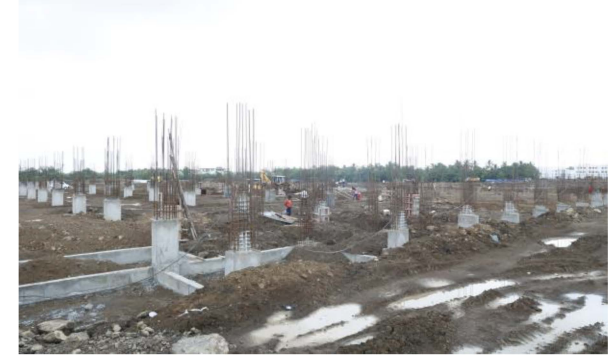
Construction going on in full swing at the 44+ acres new facility
