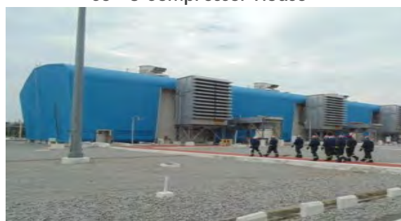
CS - 3 Compressor House
