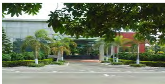
CS - 3 Local Control Room Building
