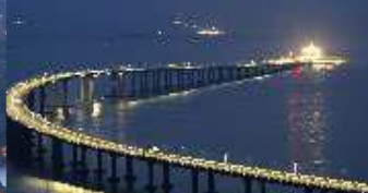
Hong Kong–Zhuhai–Macau Bridge
