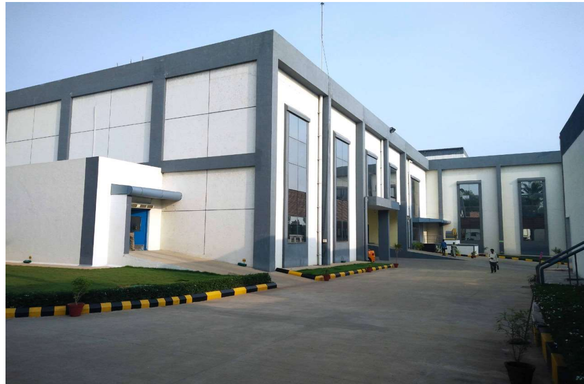
CP-I plant at Suthukeny, Puducherry
