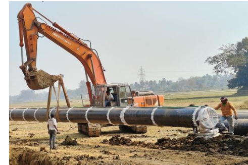
Lowering of Slurry Pipeline in Odisha
