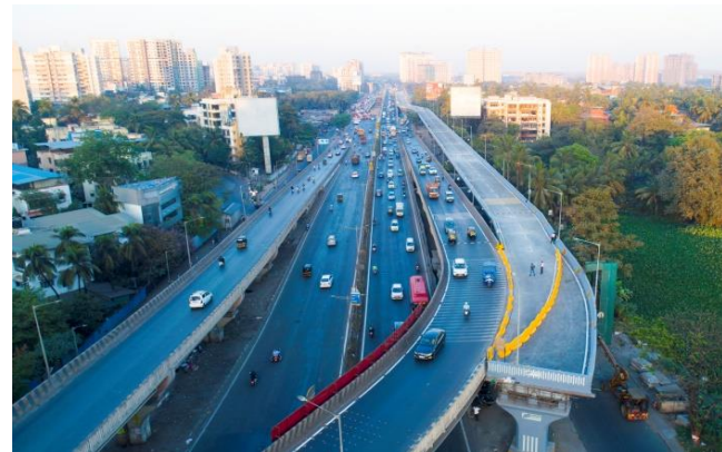
Chheda Nagar Flyover Part 1
