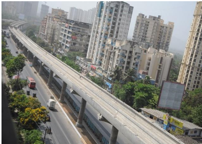
Mumbai Metro Line 4A
