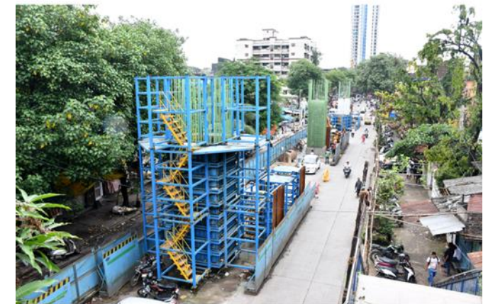
Sewri Worli Elevated
