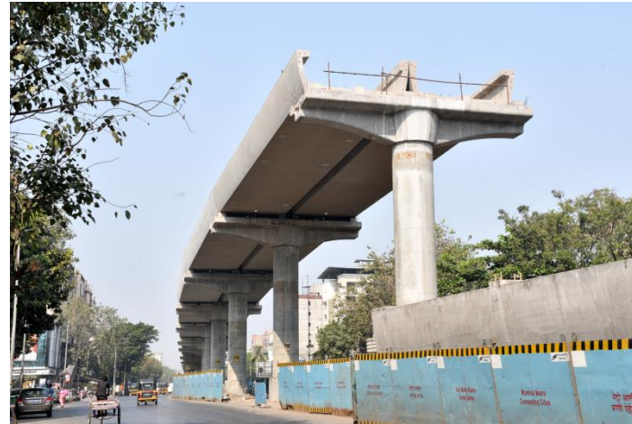
Mumbai Metro Line 9
