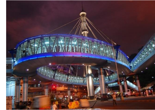
Grant road Skywalk
