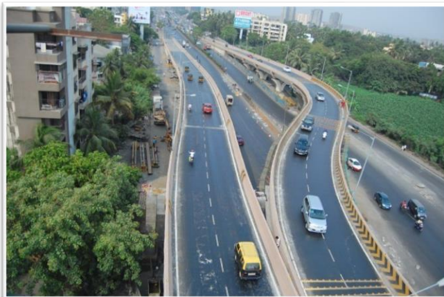
Amar Mahal Flyover
