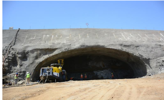
Vadodara Mumbai Expressway, IRCON
