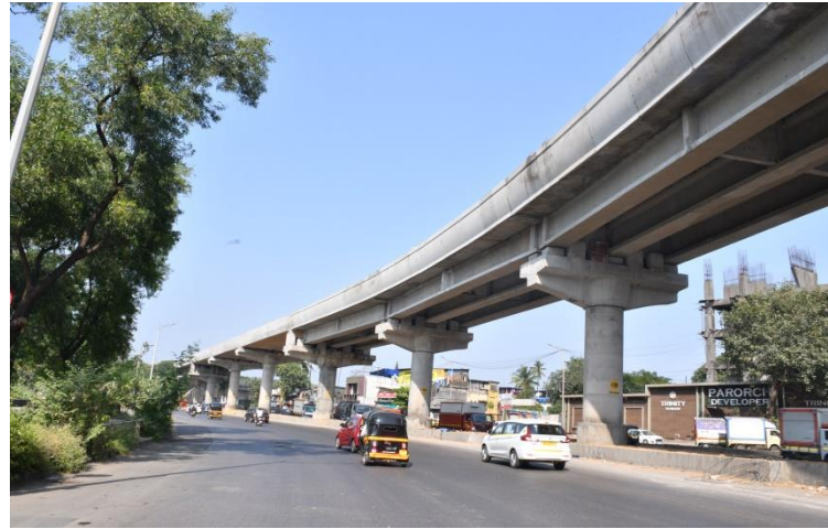
Mumbai Metro Line 6
