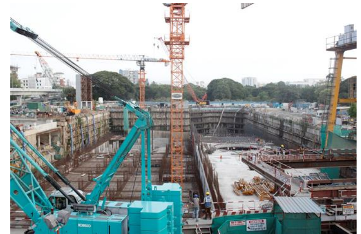
Pune Underground Metro
