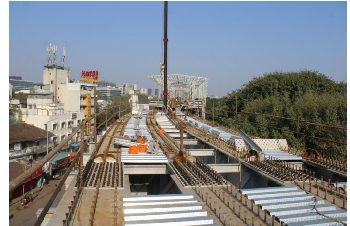
Pune Elevated Metro
