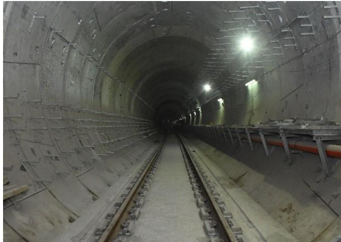
Mumbai Underground Metro Line 3
