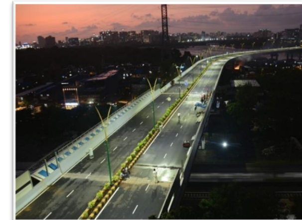
BKC- Chunabhathi Flyover
