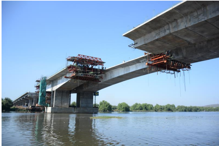
Motagaon Creek Bridge
