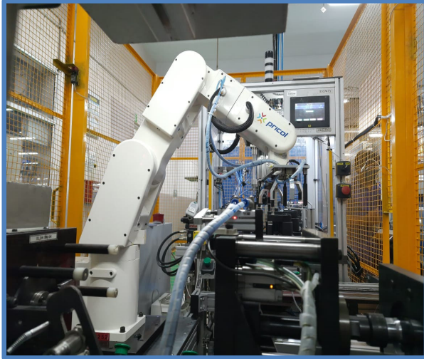
6 Axis Robot - Water pump assembly line
